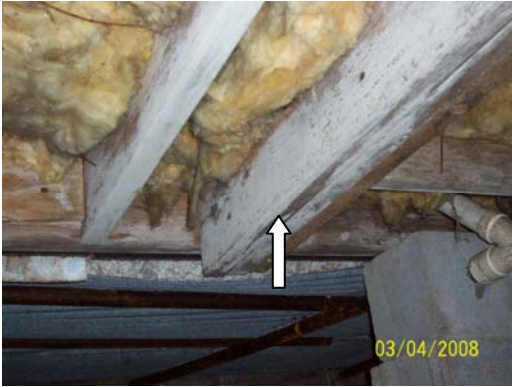
Crawlspace interior wood flooring members with fungal growth
