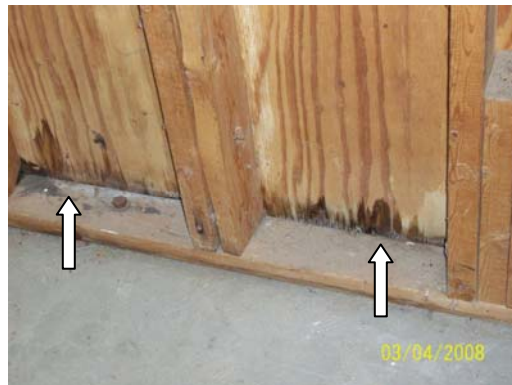
Detached garage wood siding with water penetration and peeling paint
