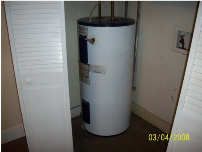
Electric water heating unit approximately 10 years of age with missing plastic PVC or copper relief valve extension tube
