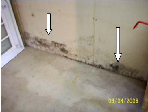
Detached garage interior wall board with heavy fungal growth
