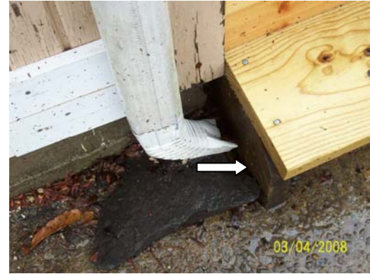
Detached garage with clogged, missing and improperly draining gutters and downspouts
