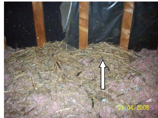
Left side attic gable vent with damaged screening and animal nesting
