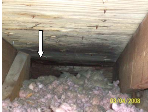
Roof sheathing with evidences of deterioration and water penetration
