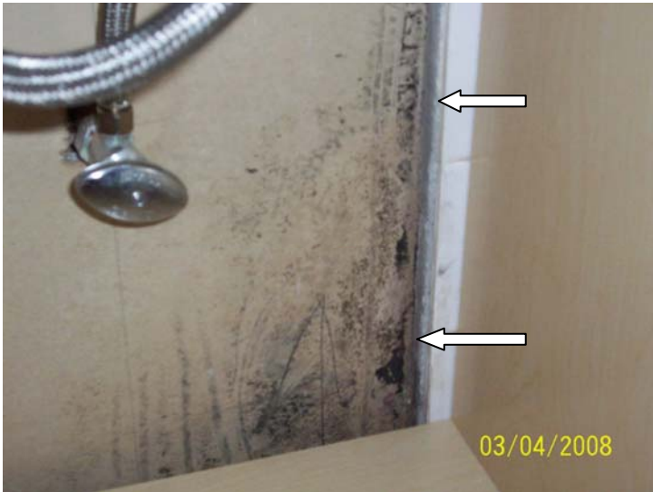
Interior master and hallway bathrooms with fungal growth on wall board located beneath sink basin
