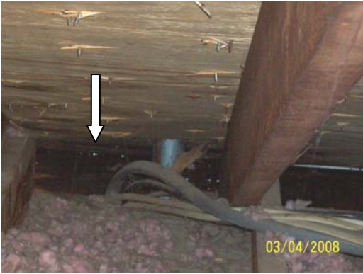
Roof sheathing with evidences of deterioration and water penetration
