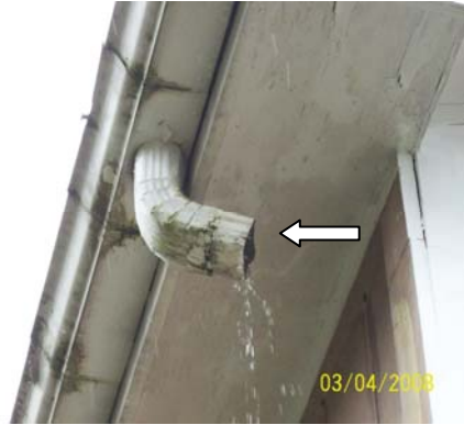
Detached garage with clogged, missing and improperly draining gutters and downspouts
