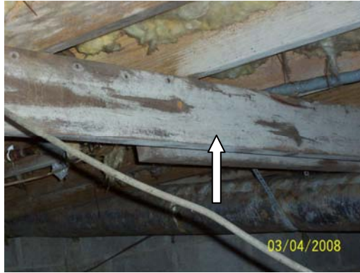
Crawlspace interior wood flooring members with fungal growth
