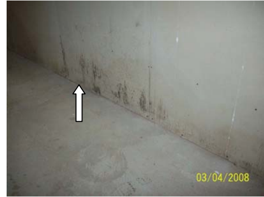
Detached garage interior wall board with heavy fungal growth
