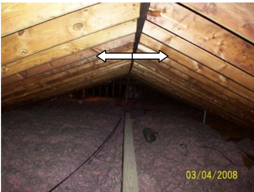
Attic roof structure with missing collar ties
