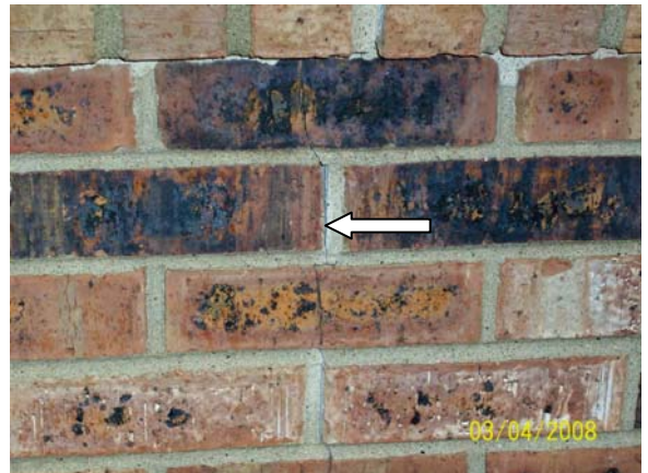
Exterior masonry siding with evidence of vertical and step cracking
