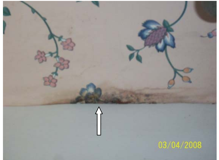
Interior master and hallway bathrooms with fungal growth on wall board located beneath sink basin
