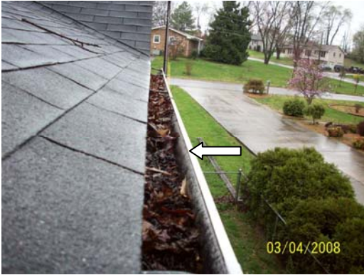
Detached garage with clogged, missing and improperly draining gutters and downspouts
