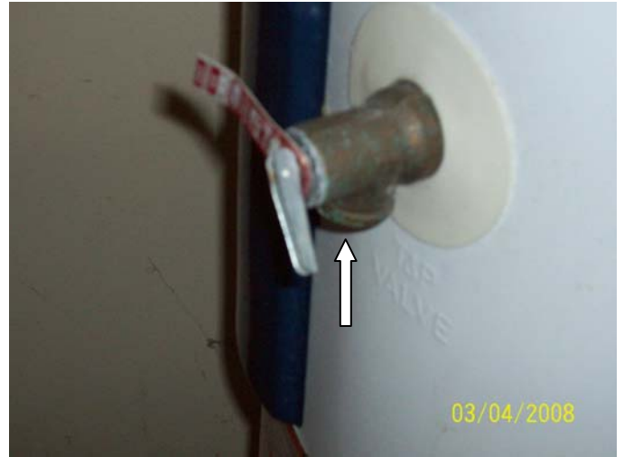
Electric water heating unit approximately 10 years of age with missing plastic PVC or copper relief valve extension tube
