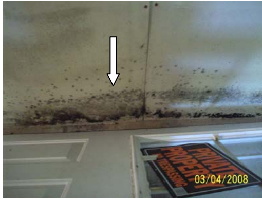
Detached garage interior wall board with heavy fungal growth
