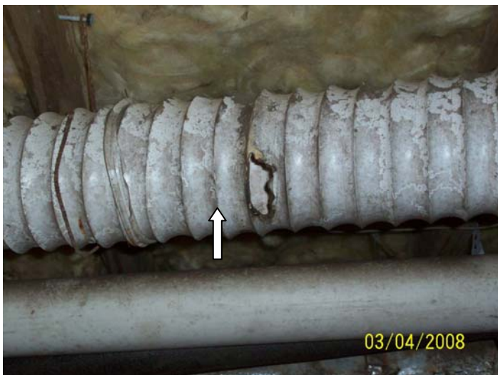
Crawlspace interior dryer exhaust hose worn and deteriorated
