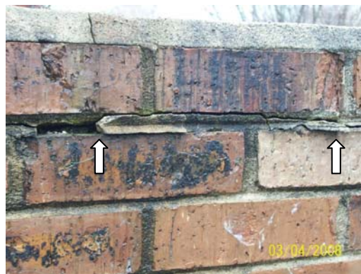
Roof chimney with spalling, deteriorated mortar joints and perimeter cracking
