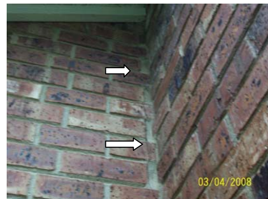
Roof chimney with spalling, deteriorated mortar joints and perimeter cracking
