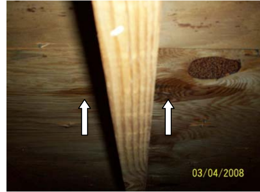
Roof sheathing with evidences of deterioration and water penetration
