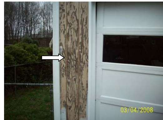
Detached garage wood siding with water penetration and peeling paint
