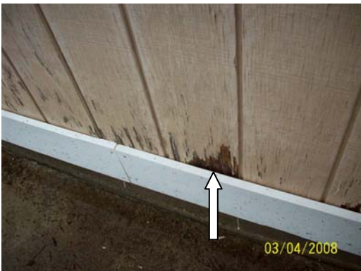
Detached garage wood siding with water penetration and peeling paint
