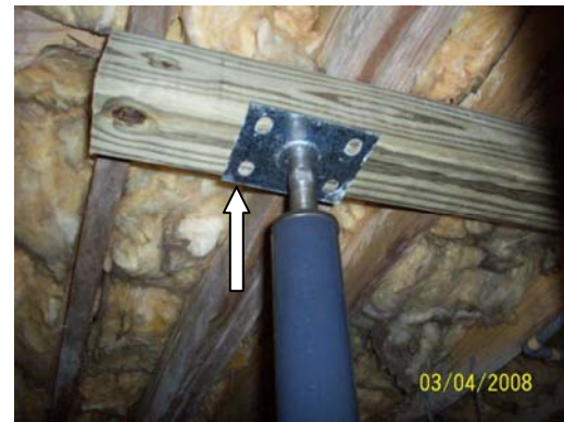
Additional support posts and 4 X 4 beam improperly installed
