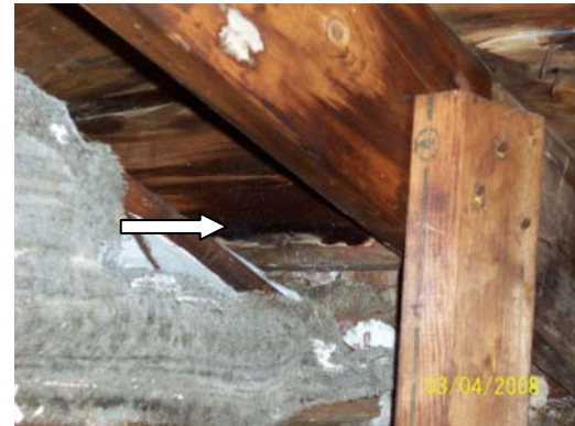
Roof sheathing with evidences of deterioration and water penetration
