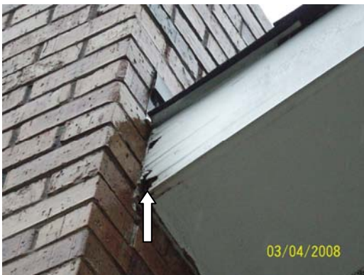
Exterior masonry siding with evidence of vertical and step cracking
