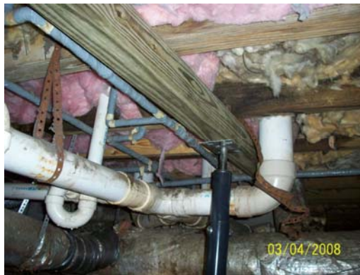
Additional support posts and 4 X 4 beam improperly installed
