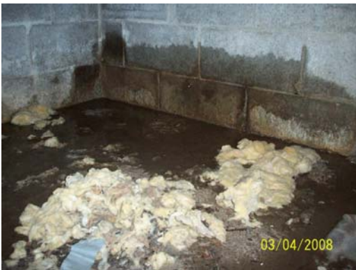
Crawlspace interior front left corner with standing water
