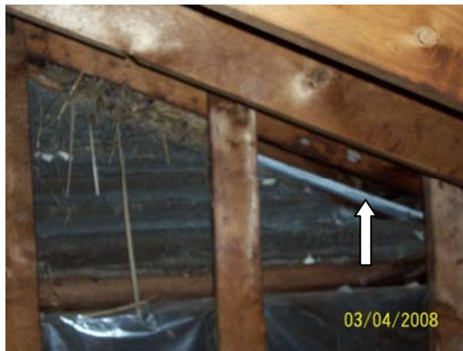
Left side attic gable vent with damaged screening and animal nesting
