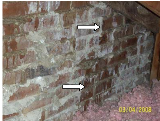
Roof chimney metal flashing leaking into the attic interior
