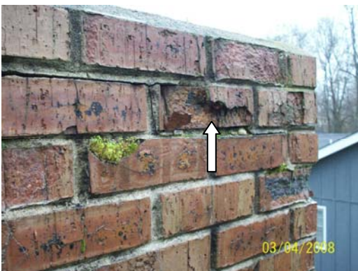
Roof chimney with spalling, deteriorated mortar joints and perimeter cracking
