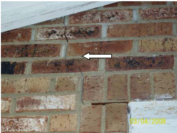
Exterior masonry siding with evidence of vertical and step cracking
